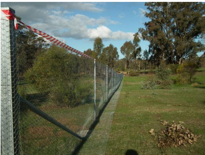
Caption: New fox- and cat-proof fencing recently installed at a protected site. (Image: B.Lobert)
